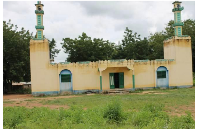
Photo 6: View of the great mosque of Broukou
